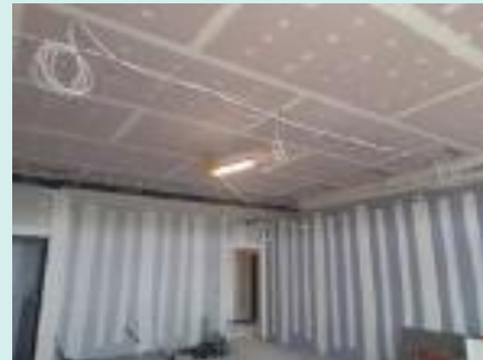
2nd. floor classroom, dry lining now completed
