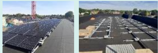
Solar Panels now being put in place.
