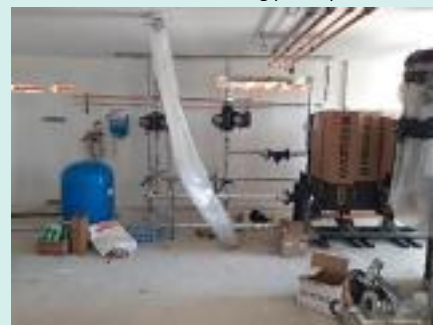
Plantroom installation in progress
