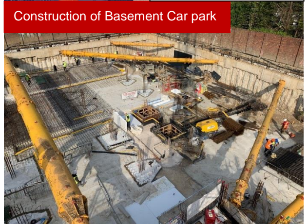
Construction of Basement Car park
